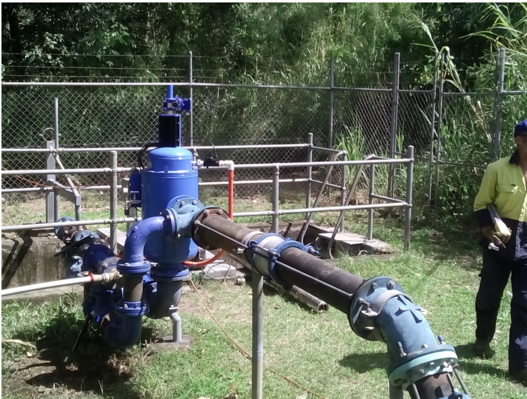
FIG 2 -1 x 100 \mu STF sintered stainless steel feed water filter at river intake.
