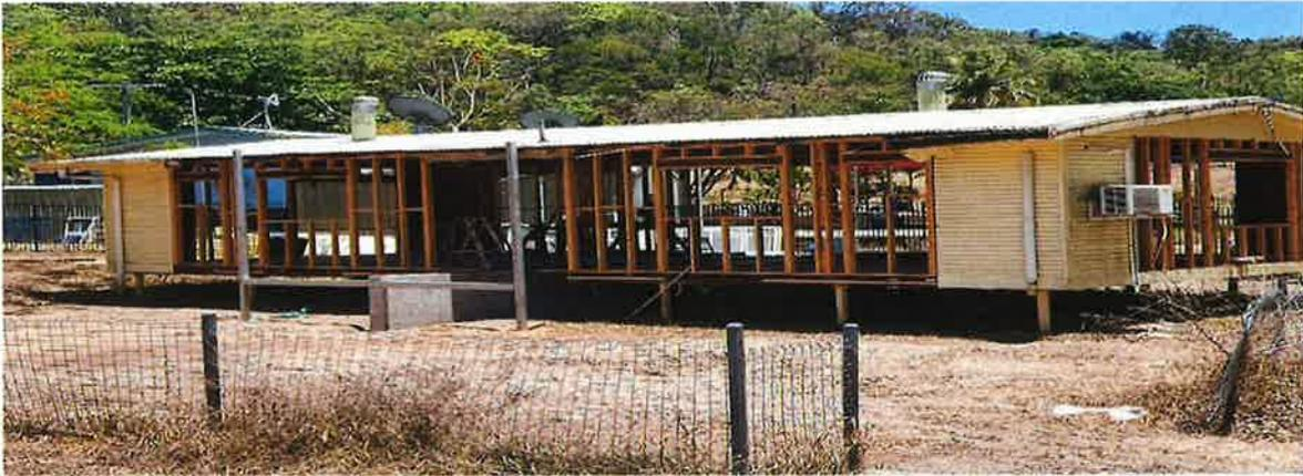
KINDY HOUSE: INTERNAL WALLS REMOVED, EXTERNAL WALLS REMOVED WHERE ROTTEN.
